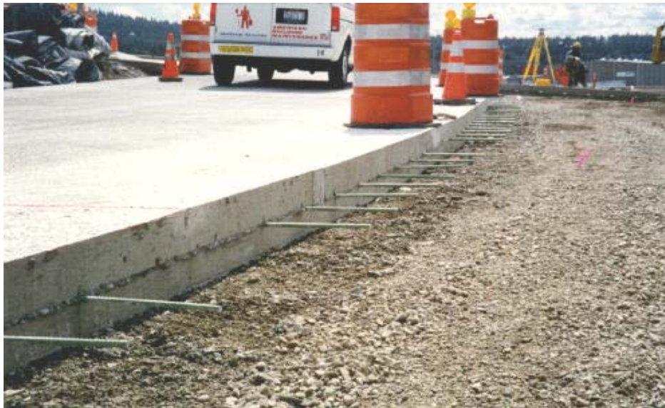
Figure 2.37: Tie Bars Along a Longitudinal Joint
