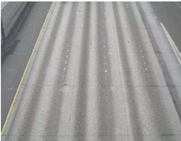
Figure 2.25: Rigid Pavement Showing Contraction Joints
