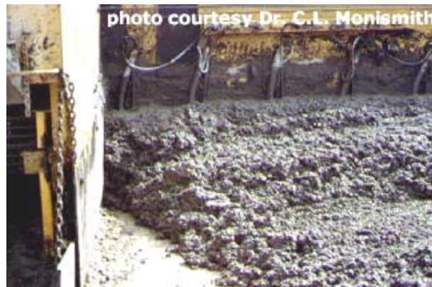
Figure 1,14: Lean Concrete Base Material
